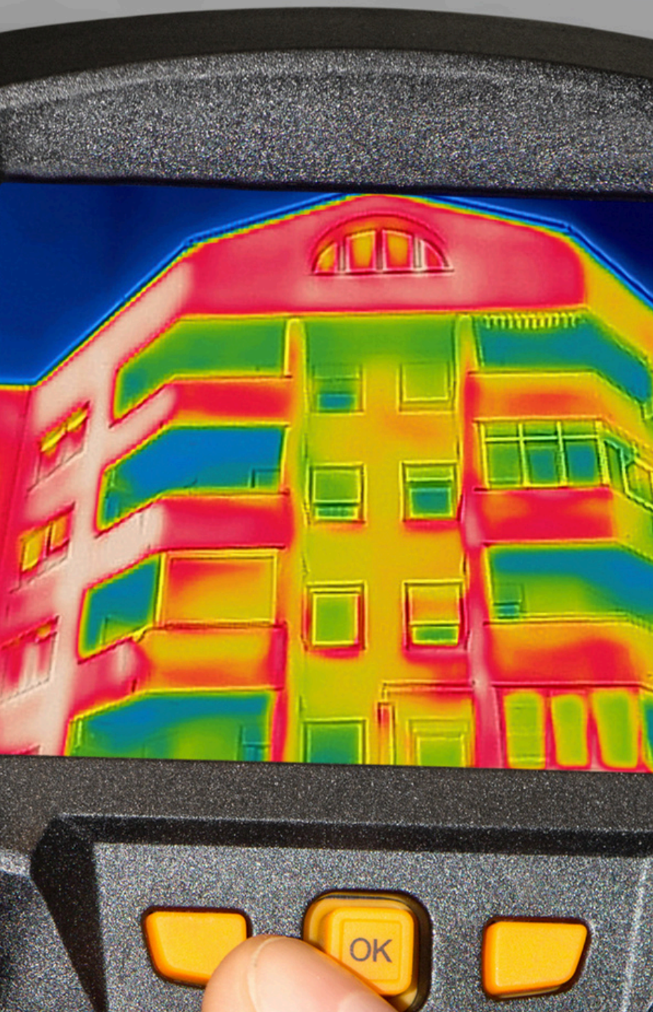
Heat loss through walls
